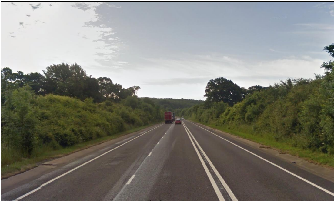
Picture 6 - Example crawler lane project on the A17 at Leadenham
