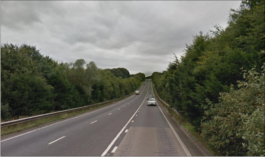
Picture 5 - Example crawler lane project on the A16 Louth Bypass
