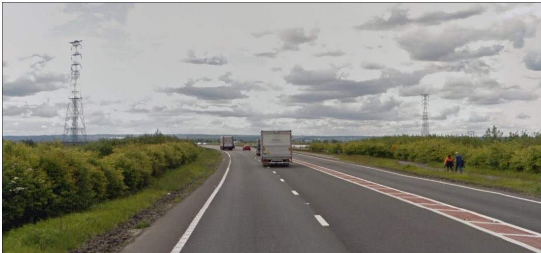
Picture 1 – Example project on the A876 to demonstrate what it will be like to travel in an eastbound direction on the A17 Gedney scheme once complete
